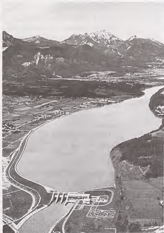
View of the Limberg Hydroelectric Power Plant in the province of Upper Austria A Drau River power plant in the province of Carinthia Courtesy Embassy of Austria, Washington
